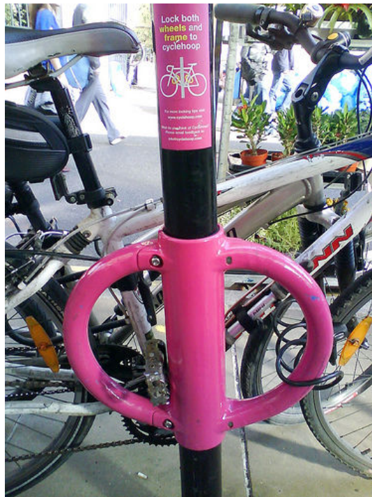
A “cycle hoop”, which is attached to existing street furniture, such as lampposts, to enable bikes to be attached securely
